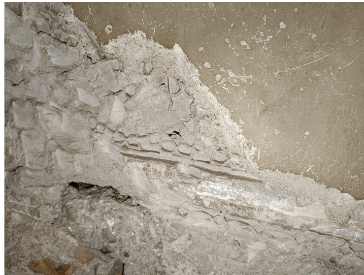
Figure 11. Fragment of plasterworks in the qibla wall. Photograph by Sergio Ramírez González.
