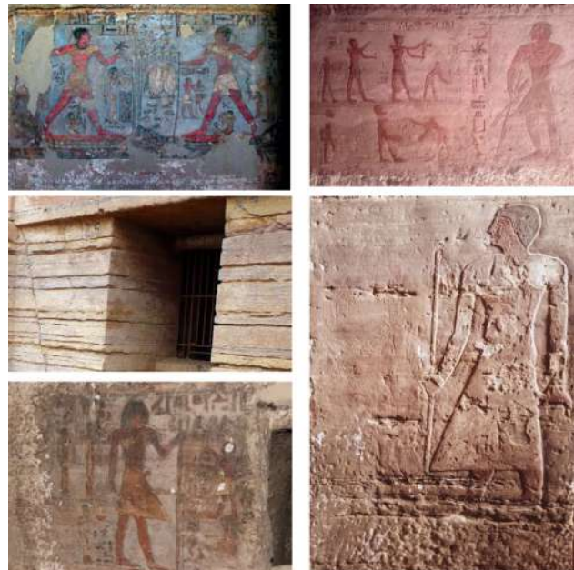
Figure 8: Deterioration of painting inside QH25 and QH26. © L. Joyanes Díaz
