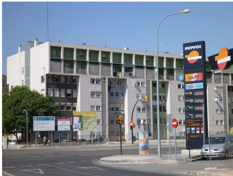
FIGURE C - 1: View of the building analysed
