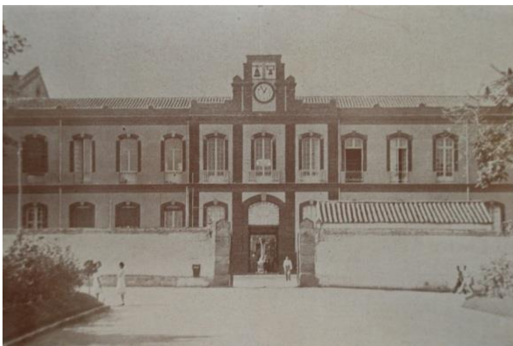
Figura 4.2 Fachada del Hospital Civil Provincial
