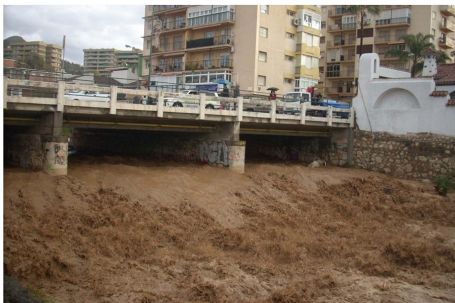
Figure 3. Photograph of one of the bridges near the Jaboneros stream mouth, after a storm, on 7 January 2010.
