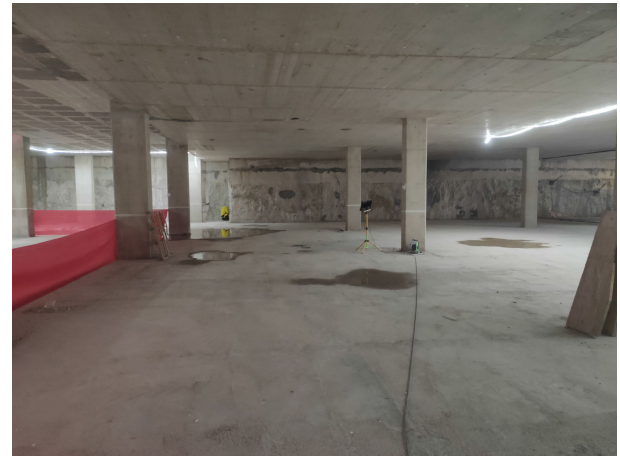
FIGURE 10. Construction scenario where the portable testbed was deployed.
