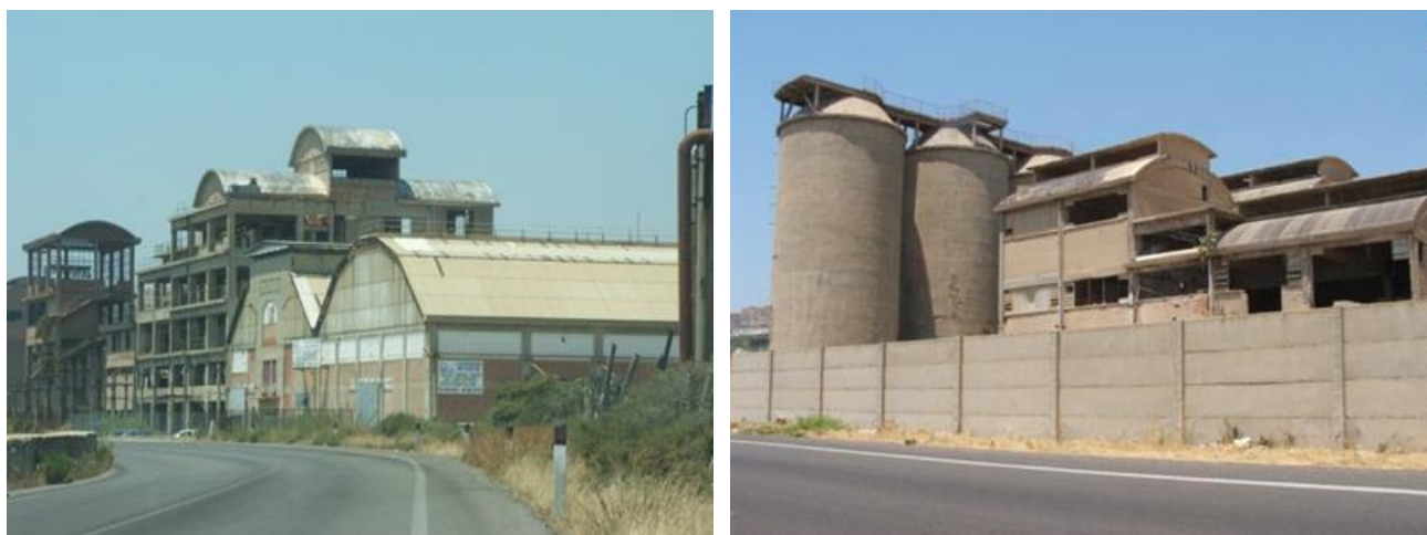
Figure 13. Potassium nitrate plant—double storage. Source: own elaboration.
