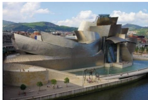
Figura 6. Guggenheim Museum Bilbao, Frank Gehry
