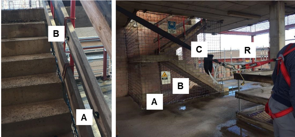
Figure 2: Two beacons are located in sequence on the side of the entry to the risk area (Left). A third beacon is located on the carabiner that connects the lifeline with the worker harness (Right).
