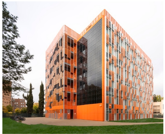
Fig. 3. Profile view “Aulario IndUVa”.
