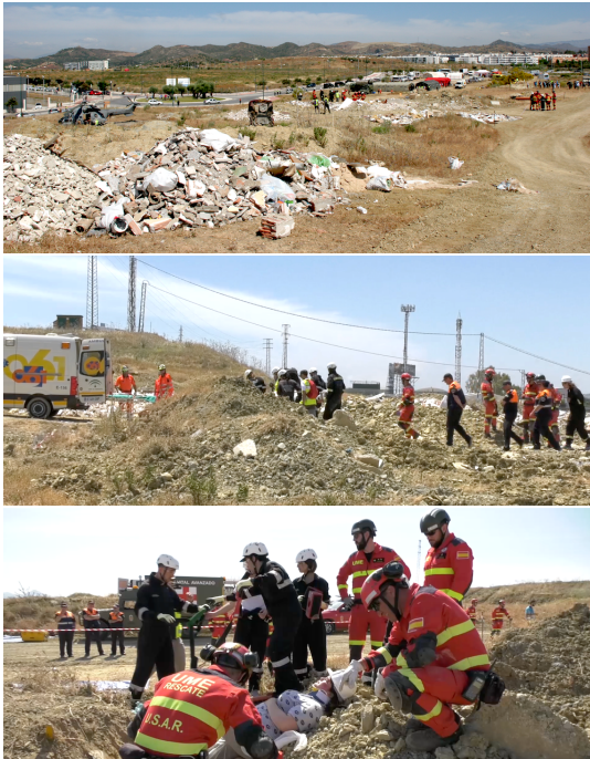
Figure 1. Photographs of the site (top) and two rescue scenarios (middle, bottom).
