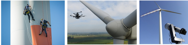
Fig. 1. Traditional types of wind turbine inspections, from left to right: manual inspection with ropes [16], drone inspection [17], and telescope inspection [18]
