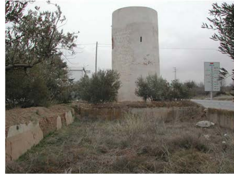
CANILES' TOWER OR TOWER OF THE MOORS
