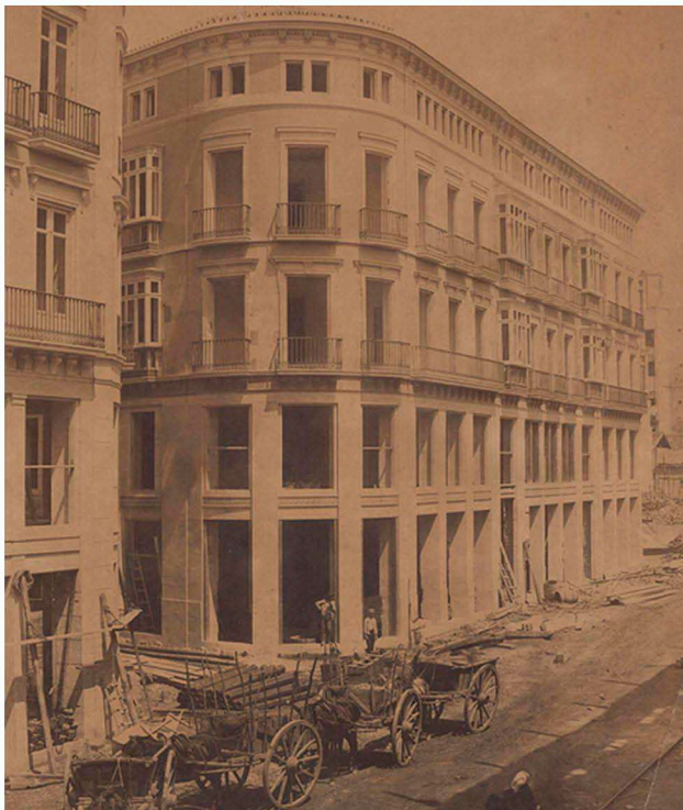
Figure 13. Building on 4 Marqués de Larios. 1889
