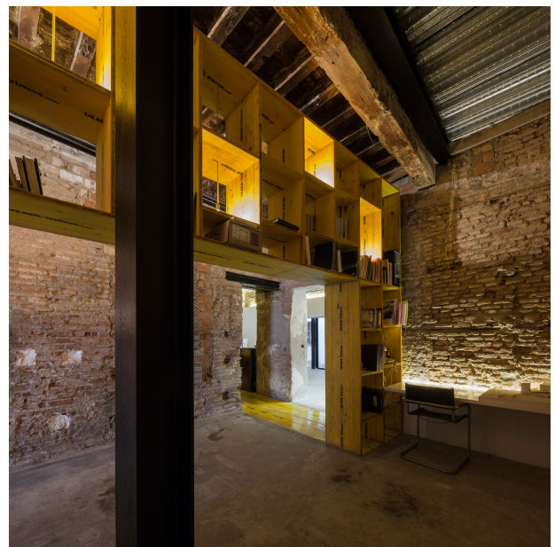
Fig 1. Atelier in San Jerónimo street, Granada: interior infrastructures insertion. Photograph: Fernando Alda
