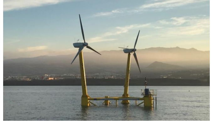
Fig. 1. Offshore wind energy semi-submersible platform W2Power concept. Image of the scaled-prototype successfully tested during spring-summer of 2019 on Canary Islands, Spain. Source: EnerOcean S.L.
