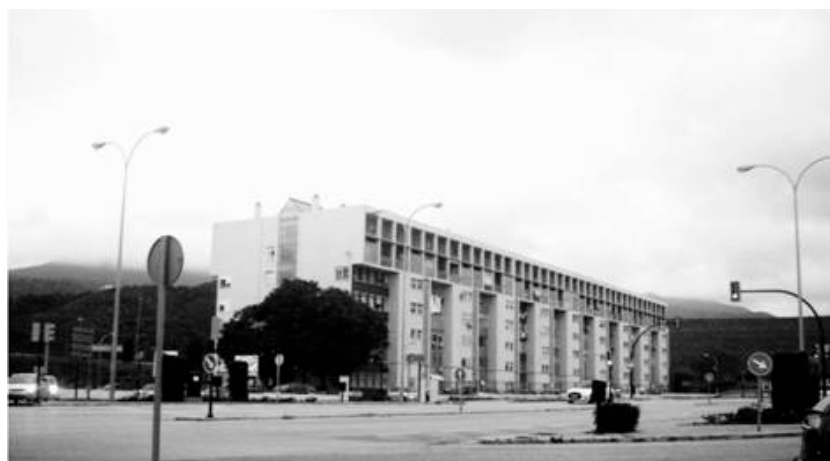
Figure 1. General view of the building.
