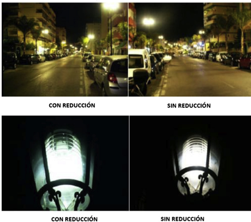
Fig. 5. Comparison of colour perception with white balance. The photographs on the left use the lighting flow dimmer-stabilizer.
